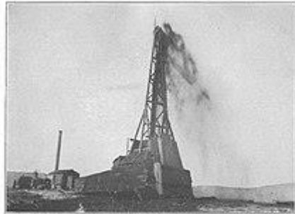
A. FLOW OF OIL AT DUTCH WELL NO. 1, DECEMBER, 1896, BEFORE WELL WAS CAPPED.
